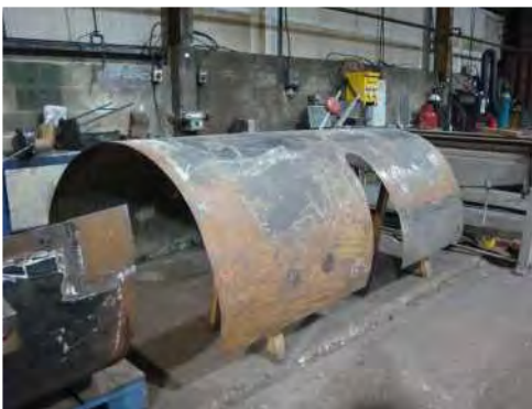
The boiler casing is undergoing repairs as necessary.
